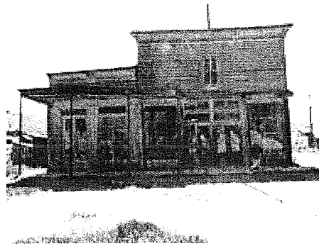
Wheaton Hollis building in Bodie. [Photo courtesy Terri Gessinger]
